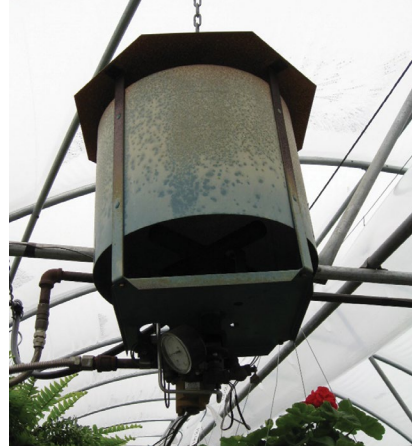
Figure 5. A carbon dioxide burner or generator burns natural gas or propane to produce carbon dioxide. Photo by Roberto Lopez.
